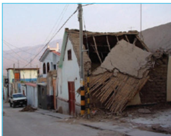
Street in Moquegua, Peru after the 2001 earthquake. Some houses appear to have little damage, but the one in front has lost its roof and may have to be rebuilt.
